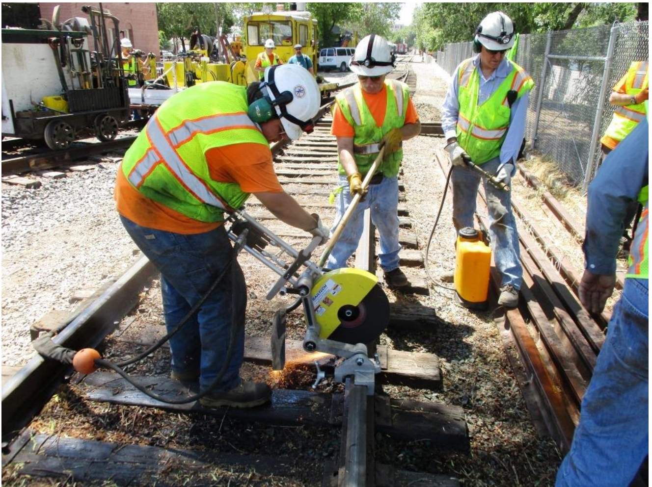
While Mike H. employs a shovel to shield sparks, Chris uses the hydraulic rail-saw to cut into the continuously-welded 113-pound rail
