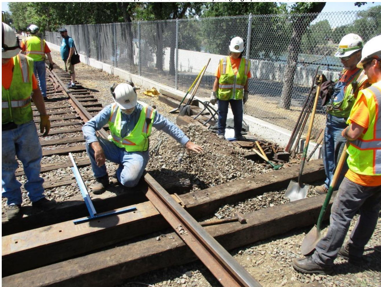
Alan uses a "t-square" to make sure everything is properly lined before securing
