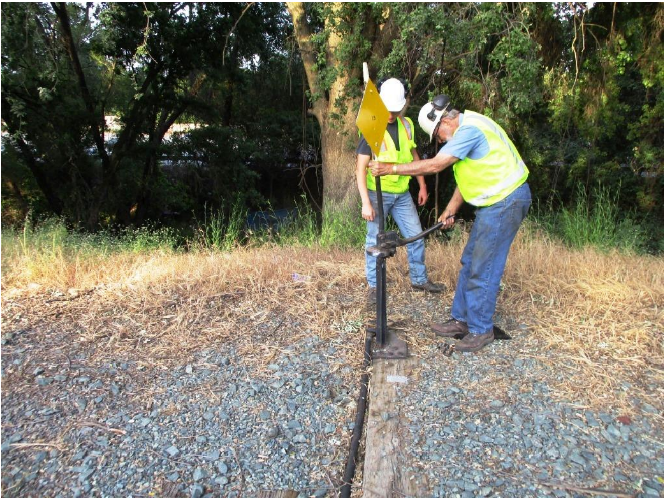
Jack and Alan make necessary adjustments to Switch 15 so that it will throw properly
