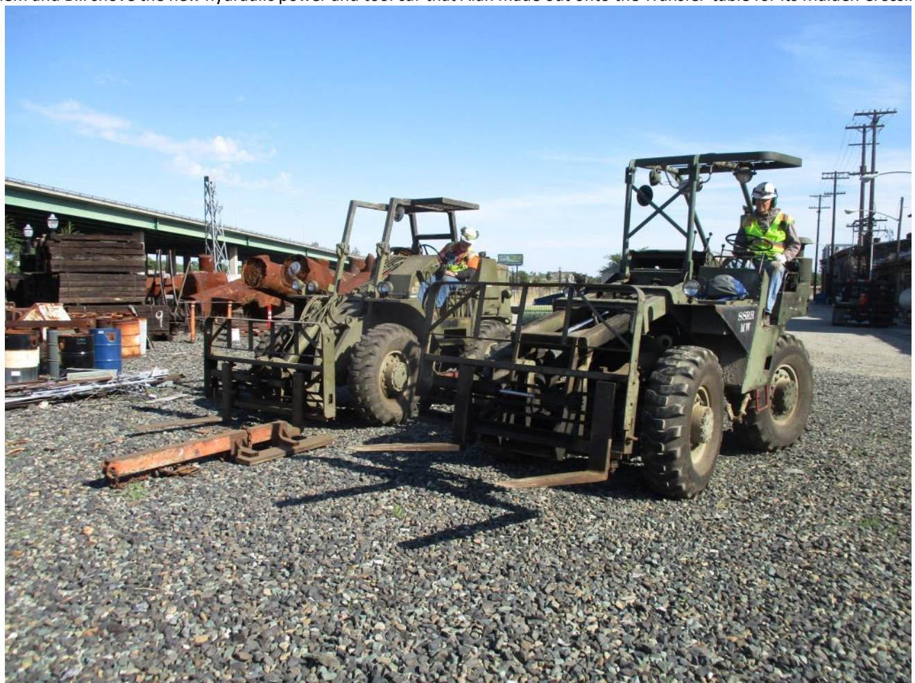
Both GM2 and Big Green were necessary to get the bevy of heavy switch components loaded onto flatcars and ready to roll
