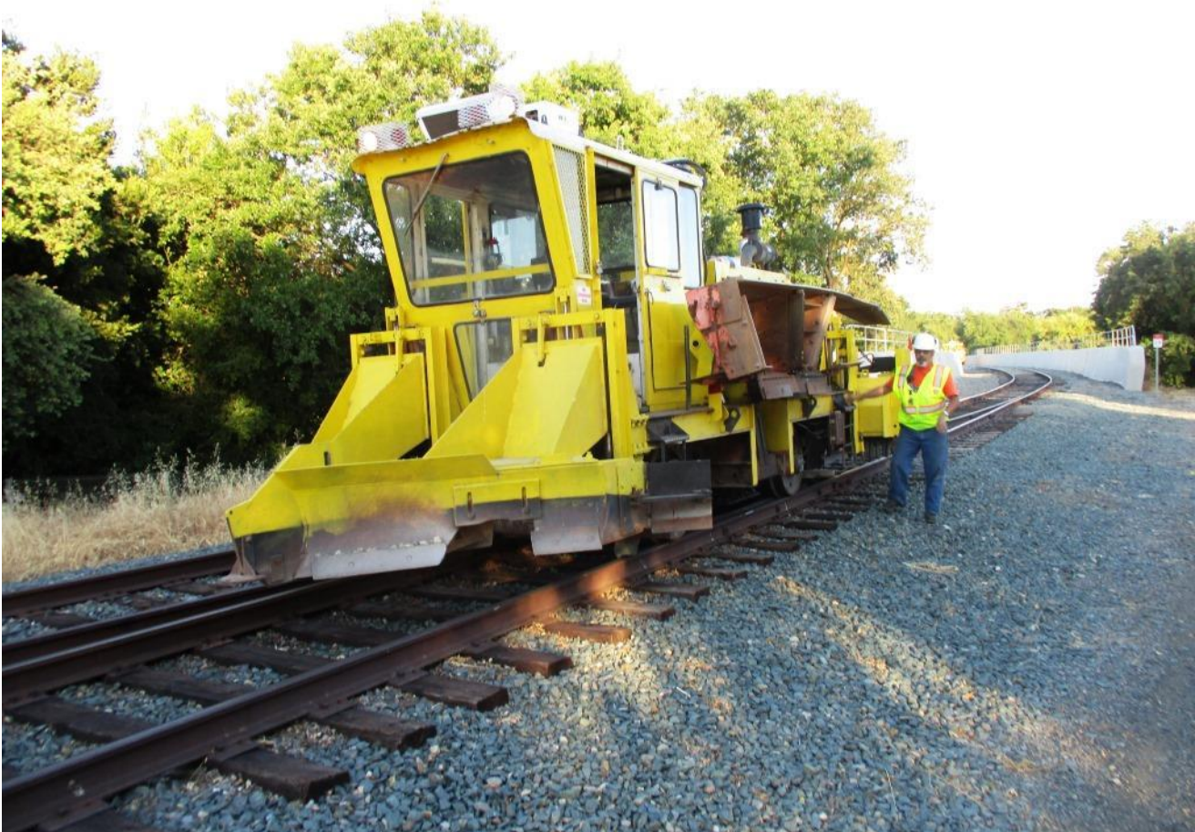
Ed with the ballast regulator ready to plow rock on the I-5 Bridge
