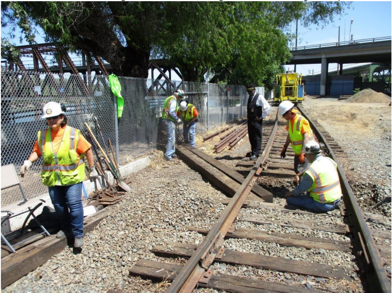
With both ties now under the rail, the real challenge is to swing them into position
