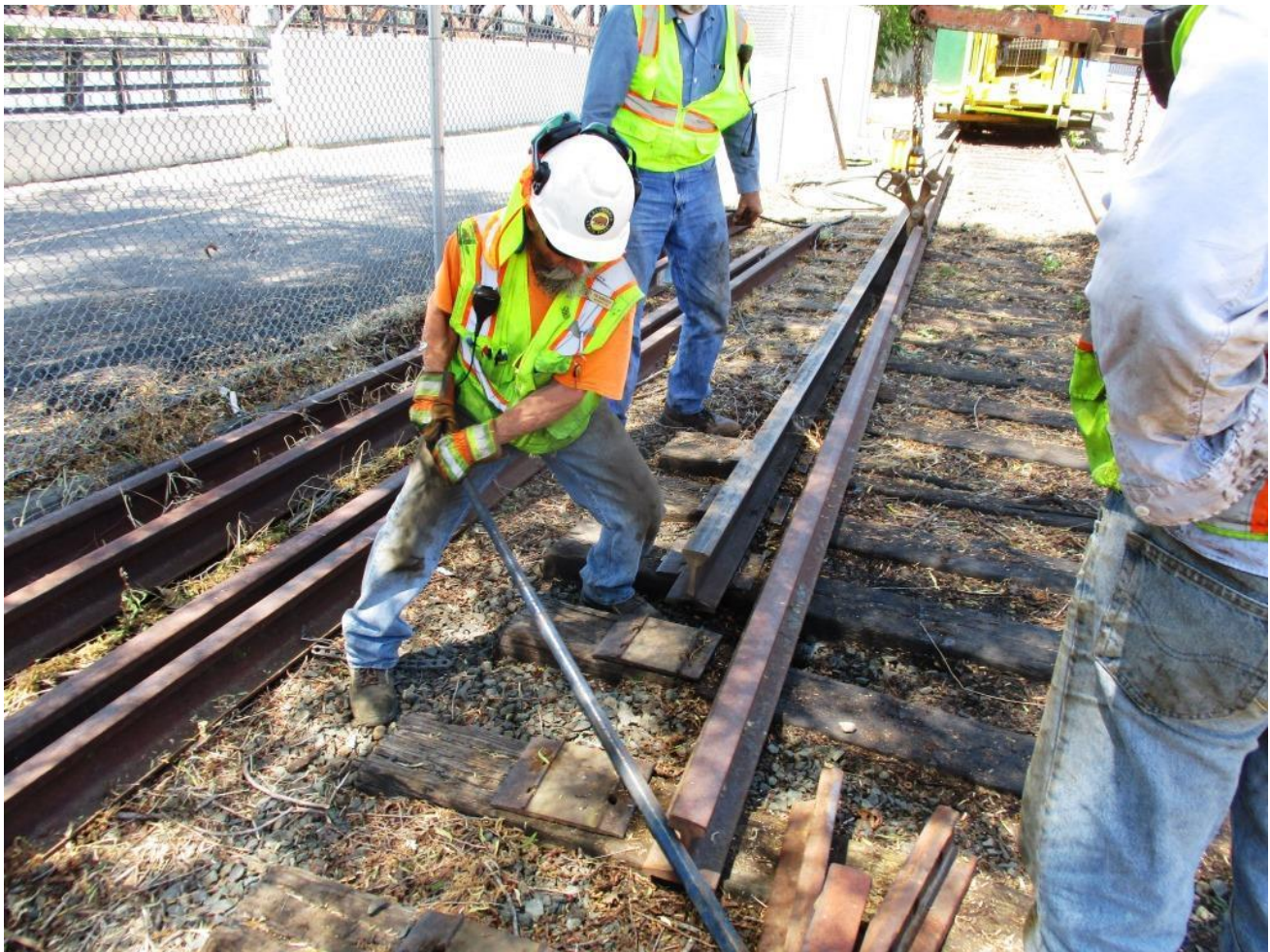
Joe uses a lining bar to shimmy the new rail into position
