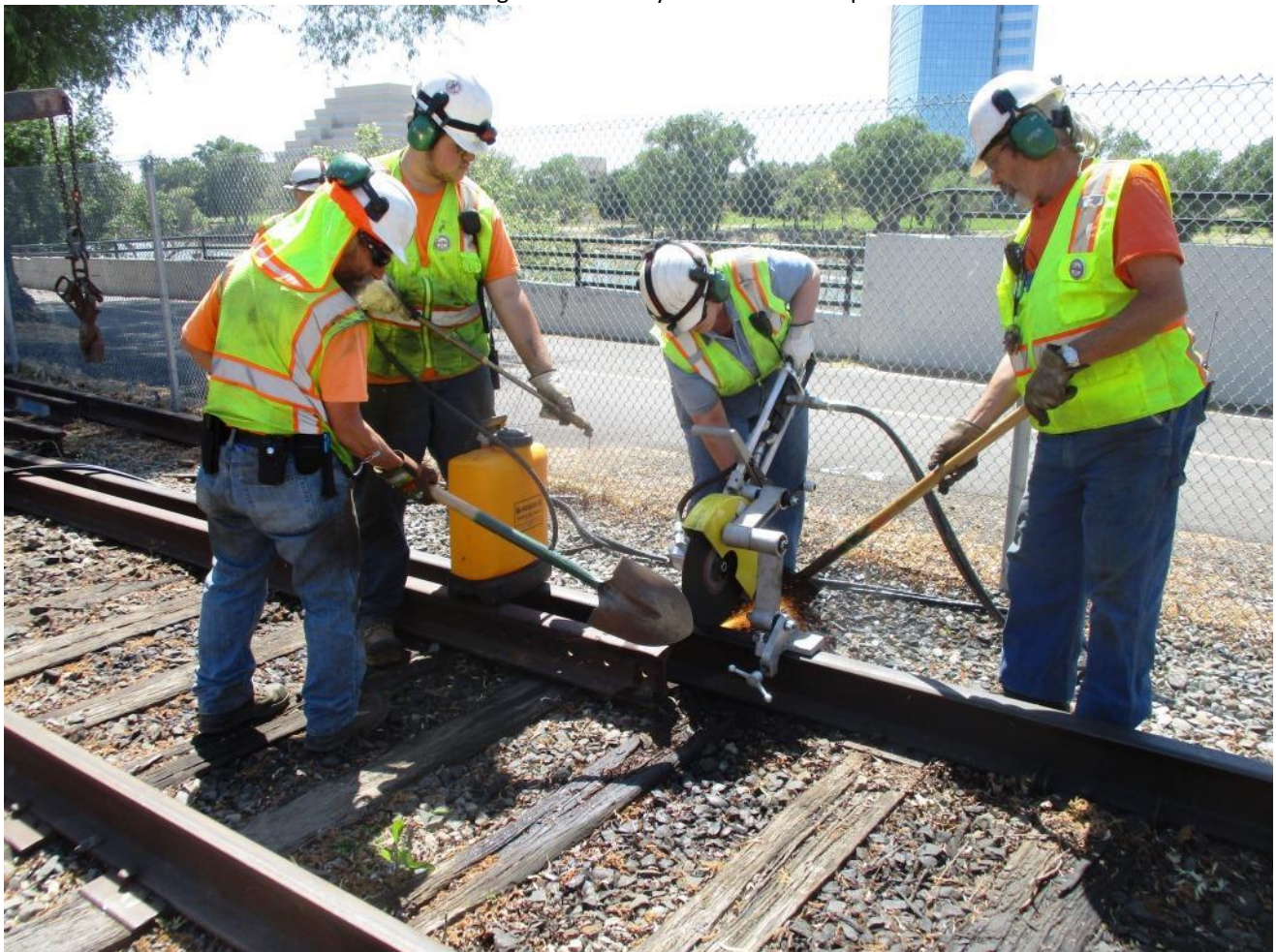
Heather makes the next cut with the rail saw
