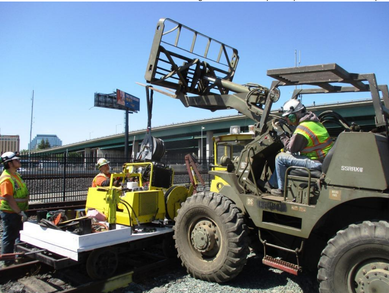
Chris and Mike F. work with Steve, now on GM2, to place the hydraulic power unit on the dedicated flatcar
