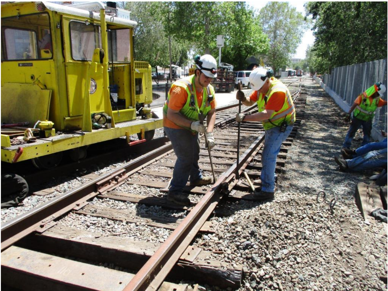
Chris and Bill tighten the bolts at the joint
