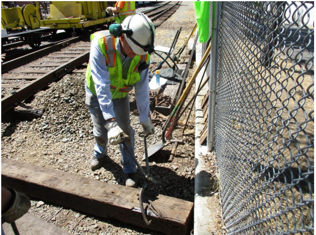
Steve grabs the west-end of the ties with tie-tongs and starts the big swing
