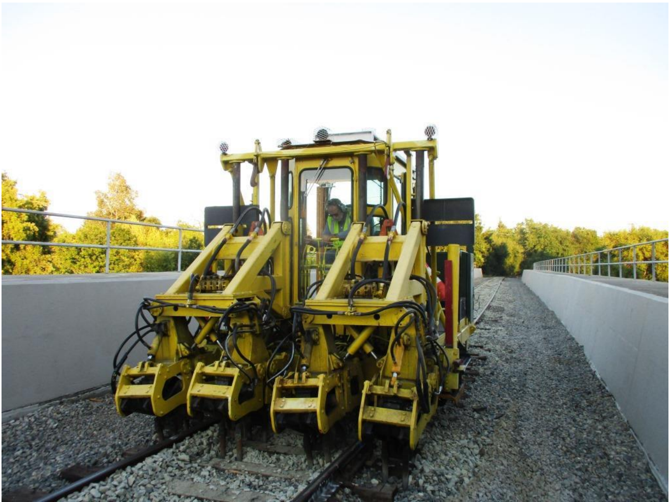
Alan tamping the I-5 Bridge track
