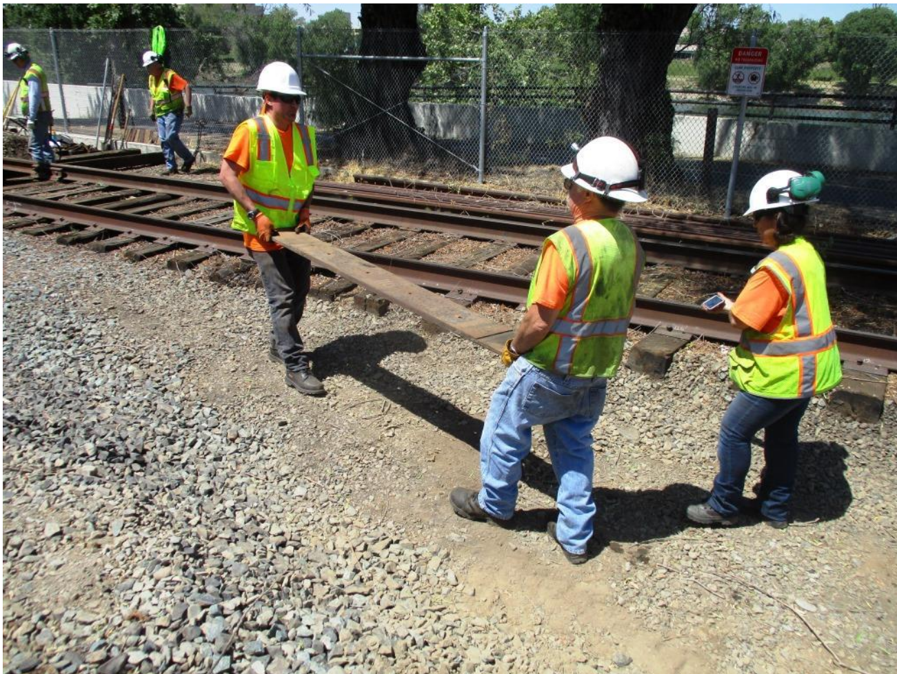
With the ties now lined-up, Hemi and Mike H. carry the gauge-plate over for installation
