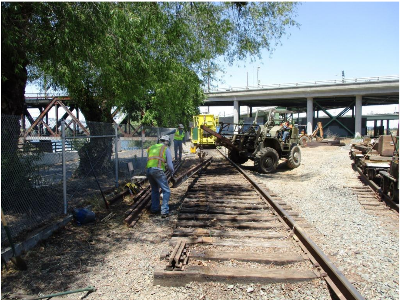
With the rail cut and out of the way, Mike F. on GM2 brings in a stick of 110-pound rail guided by Steve
