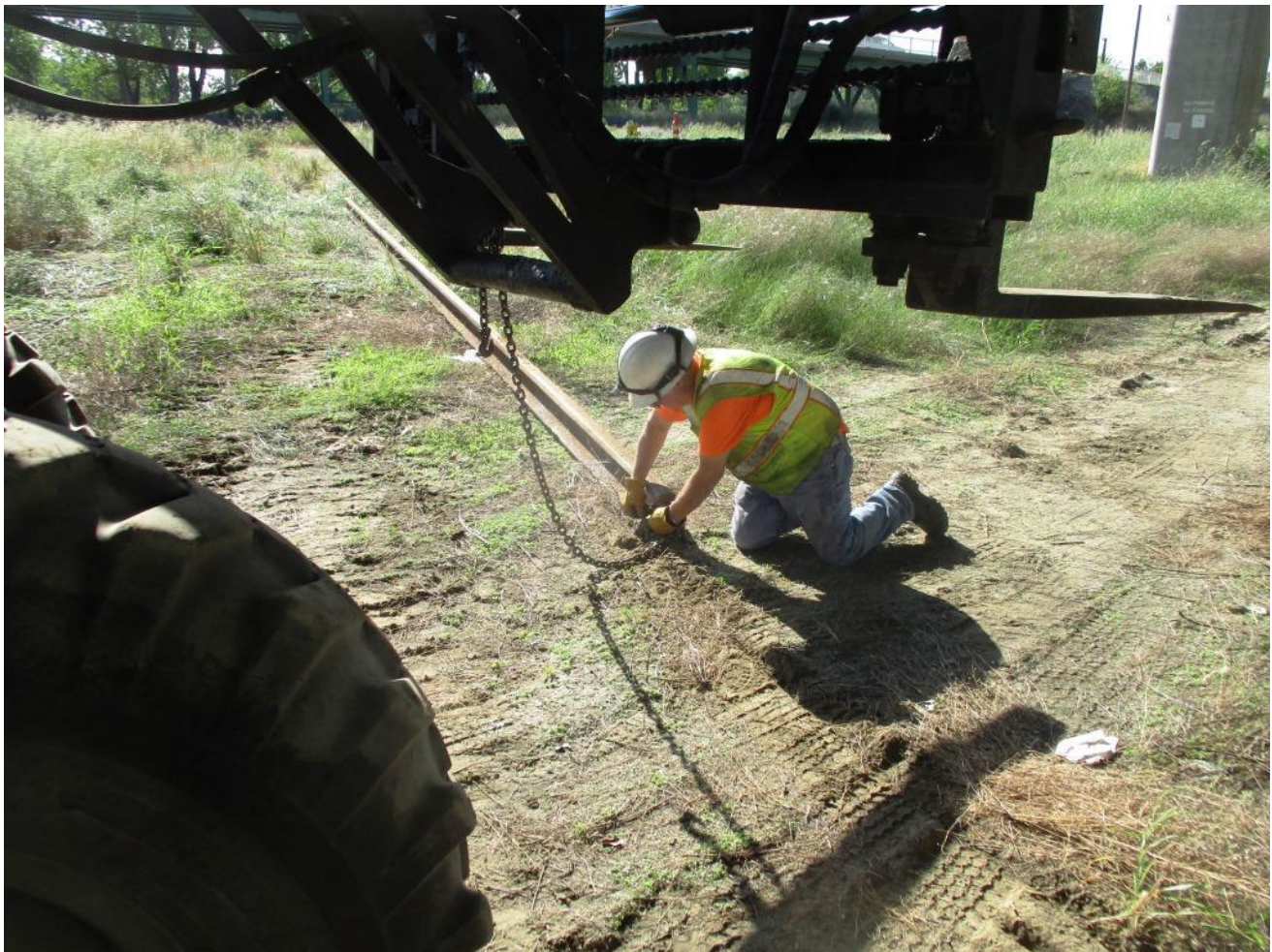
Mike H. hooks a chain to a stick of 110-pound rail which will be moved by Mike F. on Big Green
