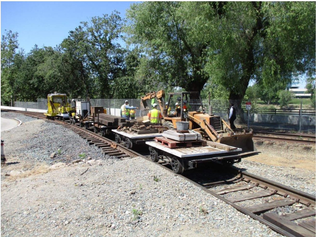
The components arrive at the job-site
