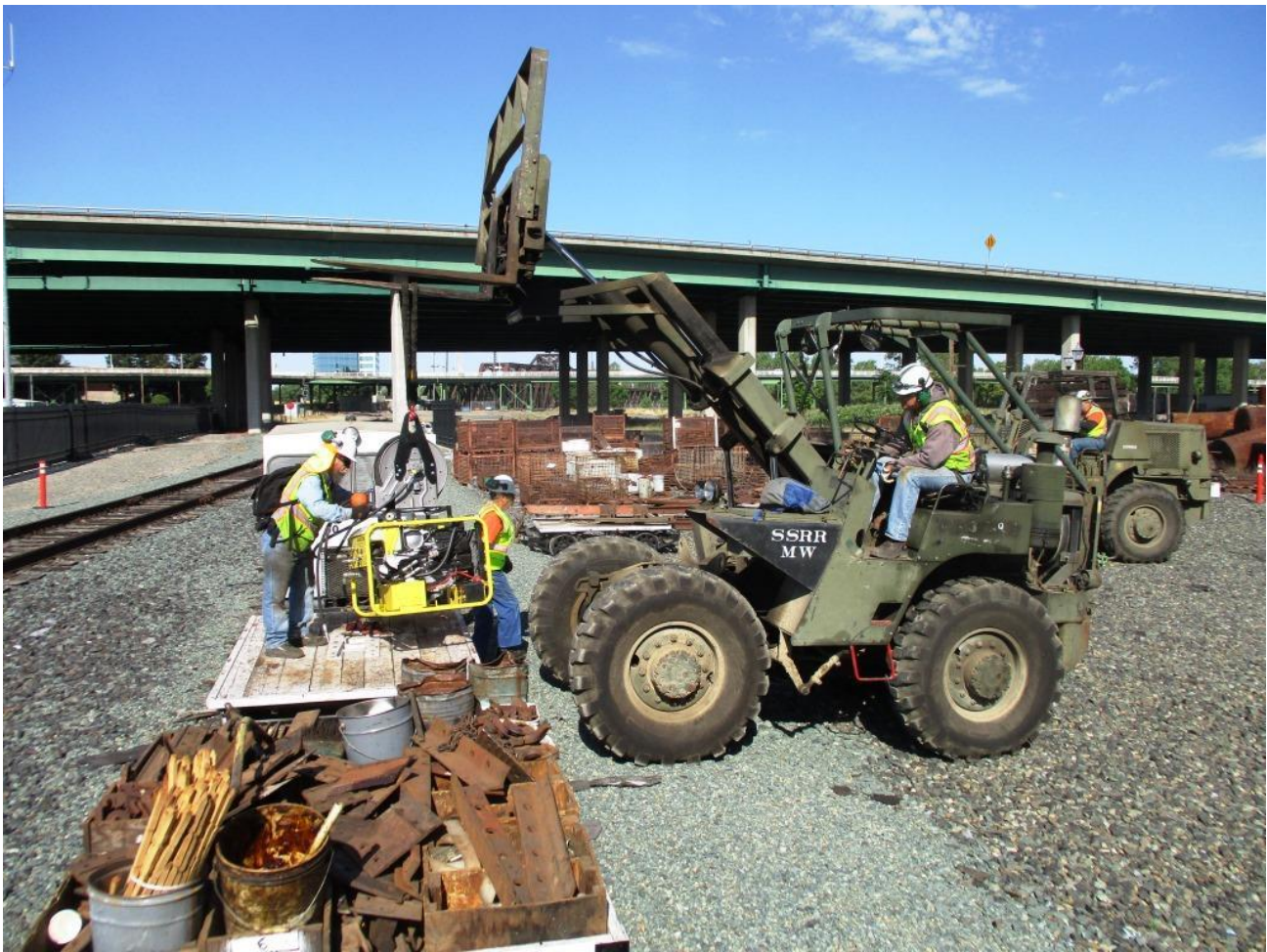
Mike F. on GM2 lifts a flatcar onto the track as Steve on Big Green moves the hydraulic power unit with Joe's help
