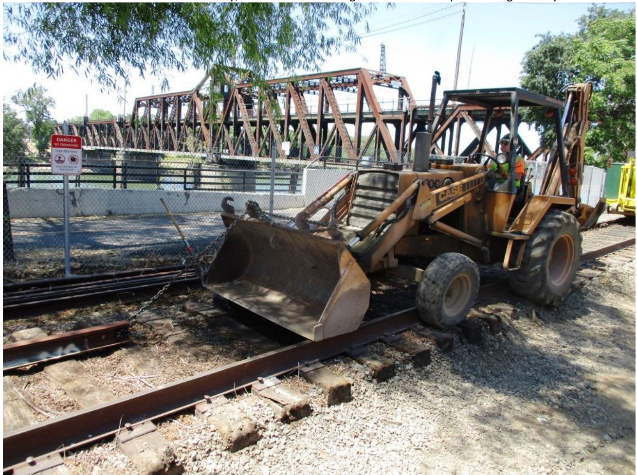
Mike H. on the back-hoe pulls the new rail into position
