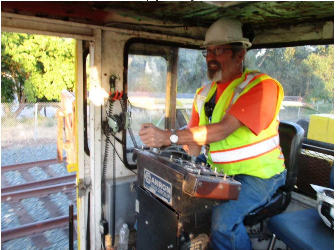
Ed at the controls of the ballast regulator
