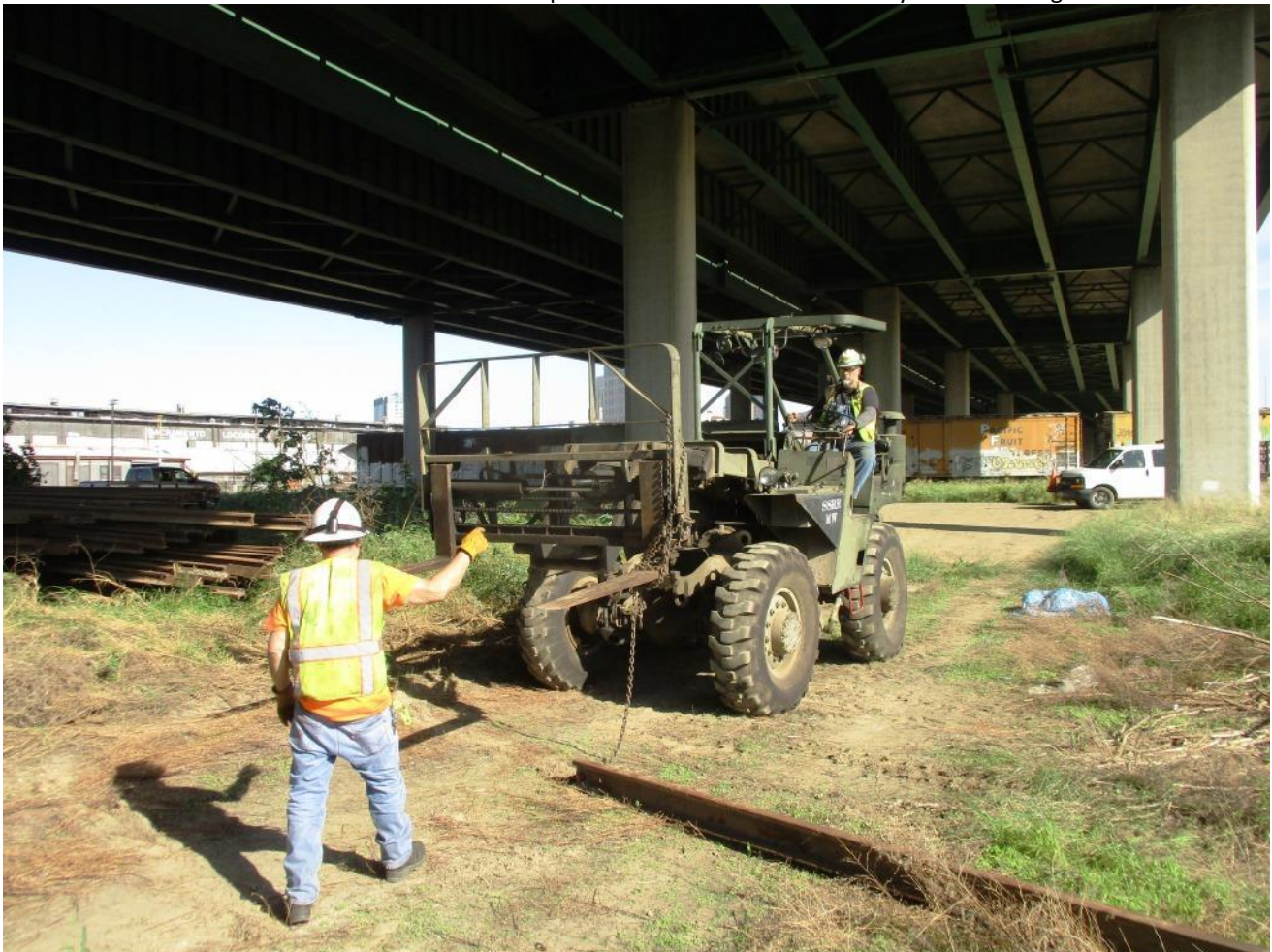
Mike H. guides Mike F. on Big Green as he pulls a stick of rail out of the pile
